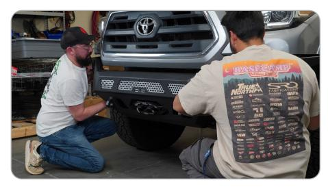
**STEP 28** Center the bumepr on the vehicle, ensuring the ends of the wings are at equal distances and heights from the headlights are equal. Usa a 14mm socket to secure the bumper in place.
